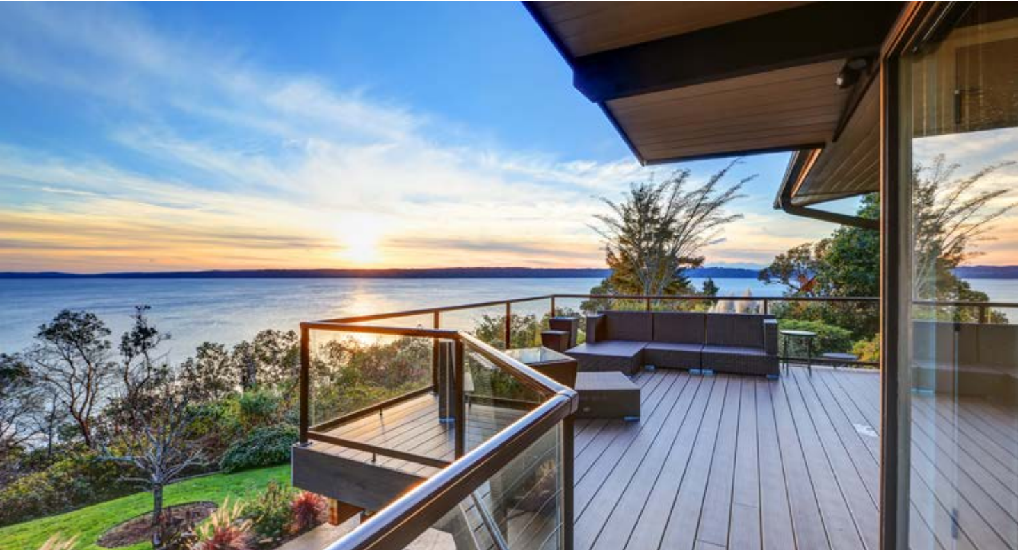
An accessible wrap-around deck allows multiple vantage points of the outdoors. Views while seated are not blocked by the handrail.
